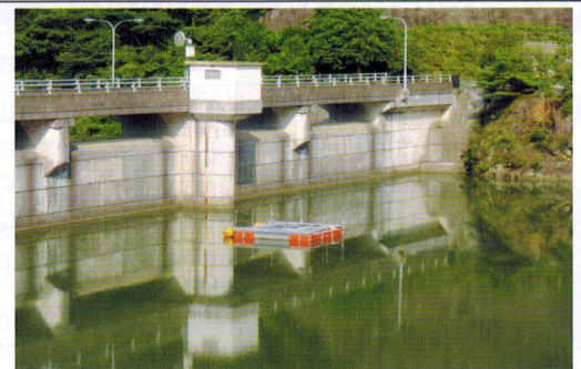
↑ Lake Controller installed in a dam lake (Motobe Dam, Saga Prefecture). The features are that it is compact and of a floating type.
